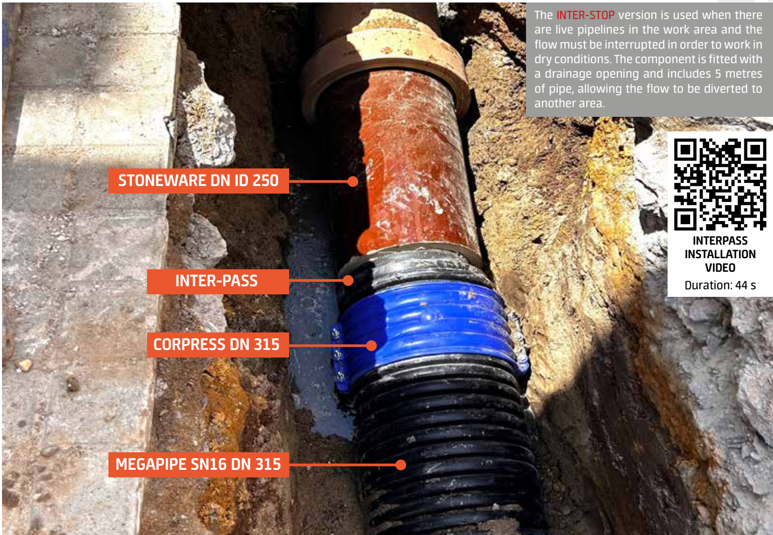
INTER-STOP WITH DRAINAGE
