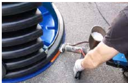
Base extrusion-welded with HDPE filler material.
