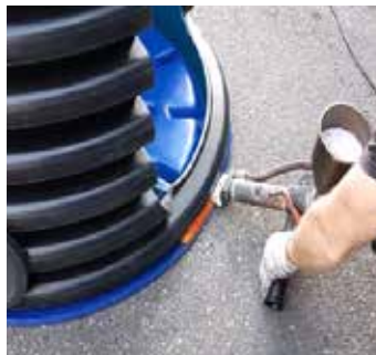
Base extrusion-welded with HDPE filler material
